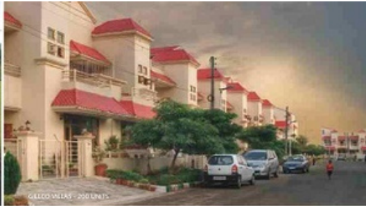
GILCO VALLEY - 250 UNITS
